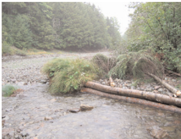
"Cumberland County River enhancement installed this habitat restoration structure on the Second River in the River Philip watershed."
