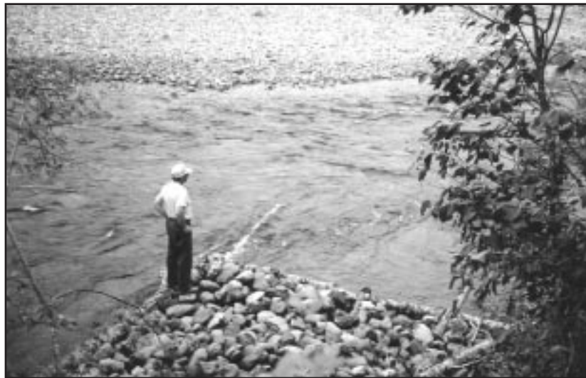
Leonard Forsyth of the Margaree Salmon Association observing a deflector working to create a pool. To date, 11 deflectors have been built in the Northeast Margaree.
