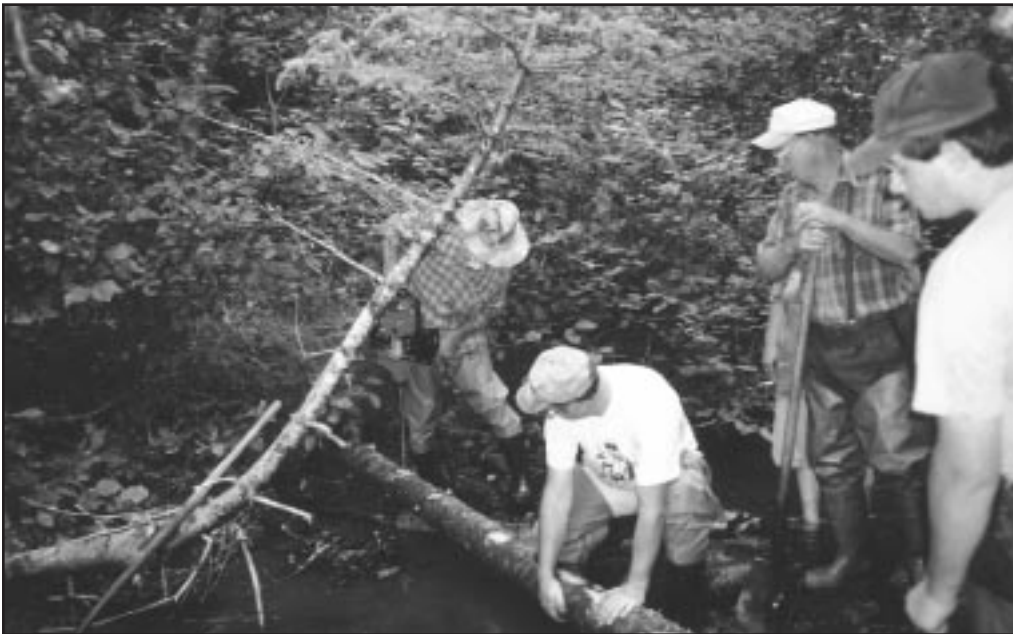
Volunteers from the Wildlife Habitat Advocates installing a digger log on French Mill Brook, Falmouth, NS
